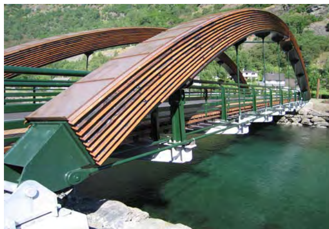
Fig. 15.17 Fretheim bridge at Flåm in western Norway (photo: R. Abrahamsen, SWECO Grøner AS)
