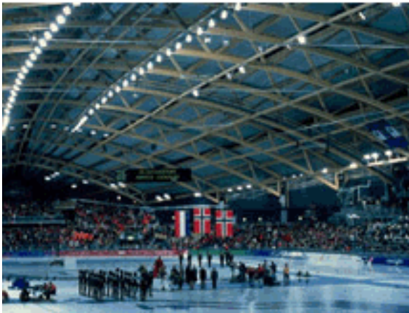
Fig. 5.14 Arches in the Hamar Olympic Hall, Norway (Reproduced by permission of Svenskt Limträ AB)
