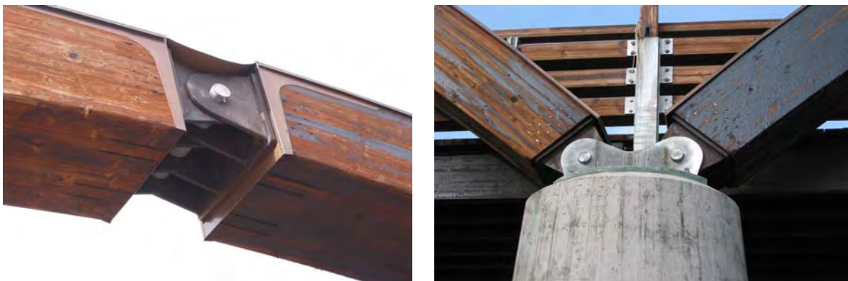
Fig. 15.14 Details of the Tynset bridge (photo: K. Bell)
