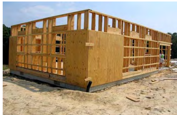
Fig. 6.6 9-layered plywood (robinia) and the use of plywood as stiffening elements in a shear-wall
