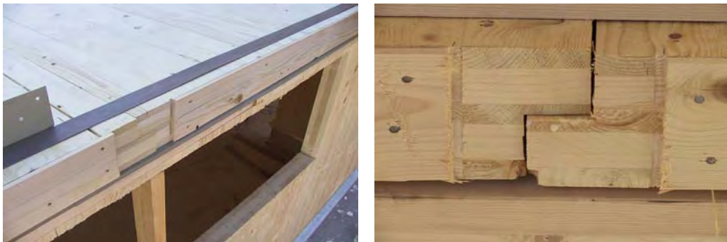
Fig. 6.38 Floor-floor-joint
