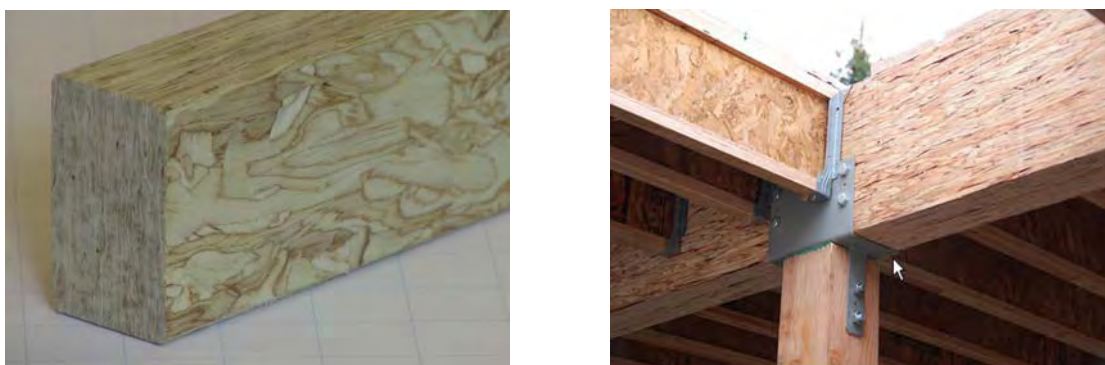
Fig. 6.4 LSL and their use as beams
