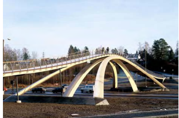
Fig. 5.5 Leonardo da Vinci Bridge in Ås, NO (Reproduced by permission of the Norwegian Public Roads Administration)
