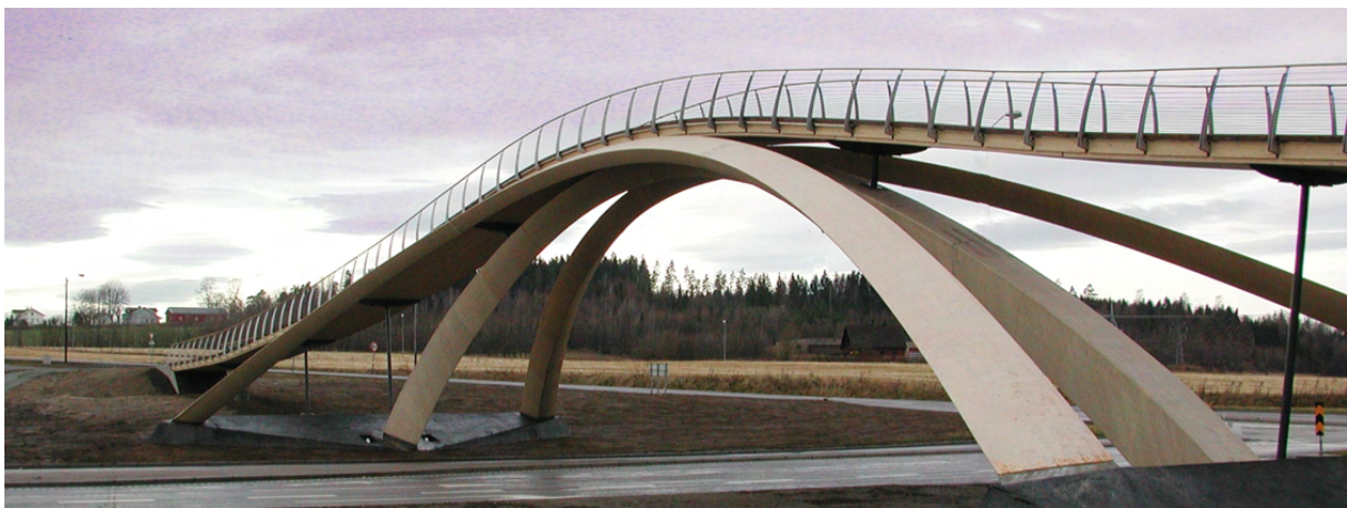
Fig. 15.2 The Leonardo footbridge at Ås, south of Oslo, Norway (photo: Moelven Limtre AS)
