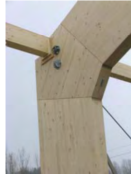
Fig. 10.5 Finger-joint of a glulam lamella and glued frame corner
