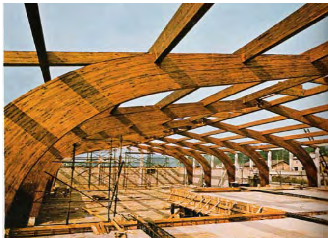
Fig. 11.3 Example of a glulam arch
