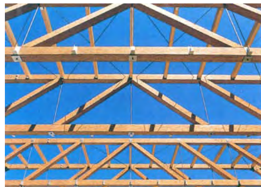
Fig. 6.5 Parallam and its use as chords in a truss
