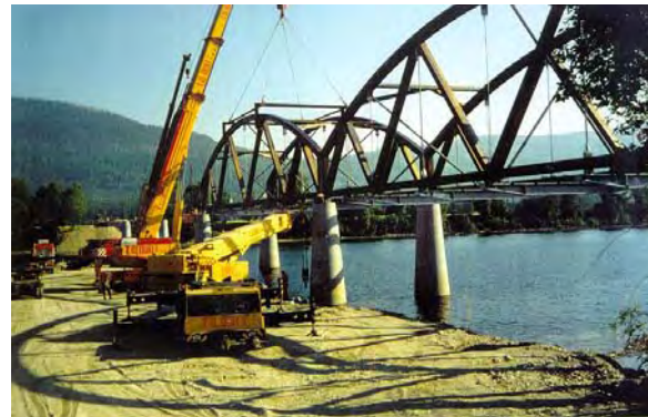
Fig. 15.18 Erection of Evenstad bridge in 1996 (photo: Moelven Limtre AS)
