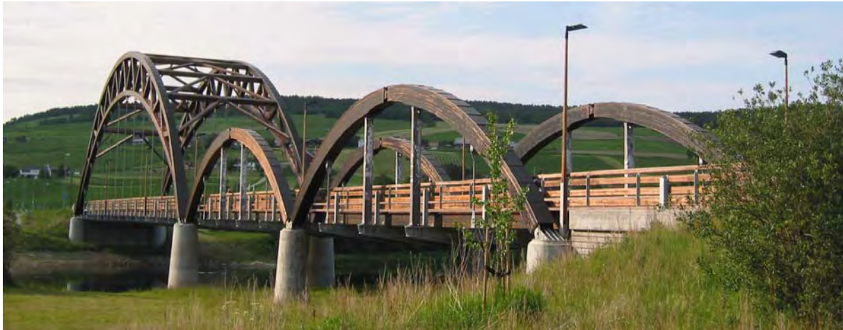
Fig. 15.6 Tynset bridge, Norway (photo: K.Bell)
