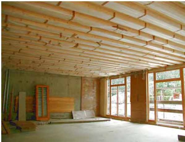
Fig. 6.34 Ribbed plate and boxed cross-sections built-up with CLT-elements
