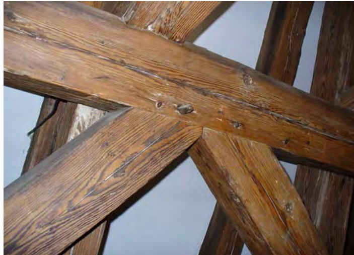
Fig. 9.6 Carpentry joints
