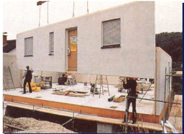
b. Mounting of walls on the building-site
