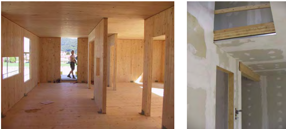
Fig. 6.30 Load-carrying elements and shear-walls in a multi storey building; floors with openings
