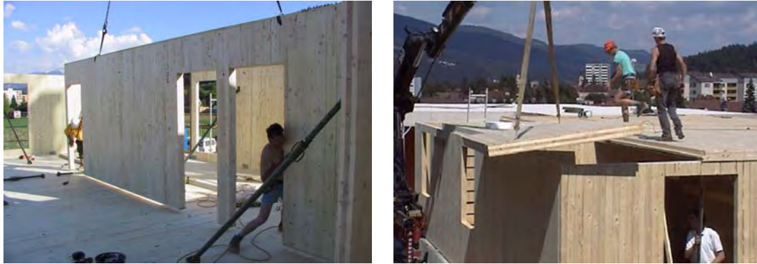
Fig. 6.29 Unfinished building: Erection of walls, lifting of floors
