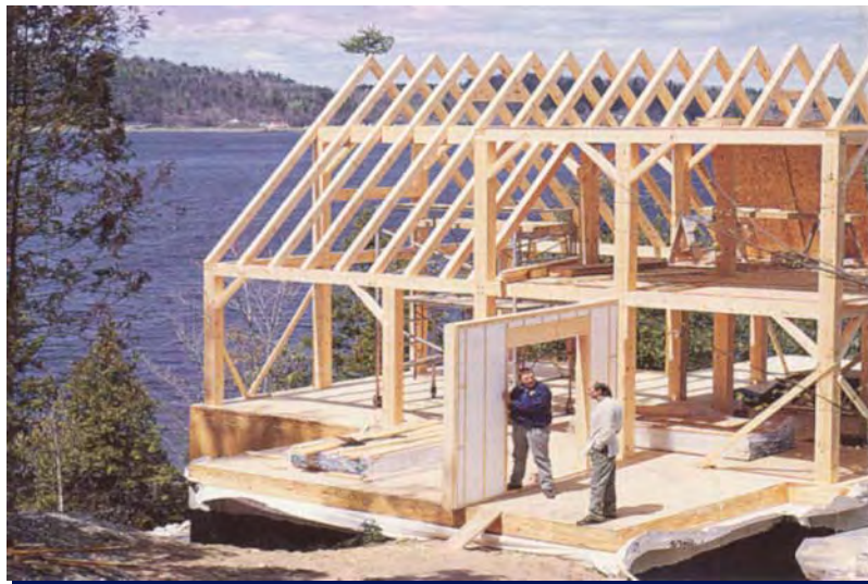
Fig. 13.1 Post and beam building system
