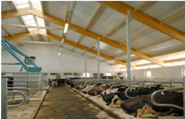
Fig. 5.10 Three-pin frame in a barn in SWE (Reproduced by permission of Svenskt Limträ AB)
