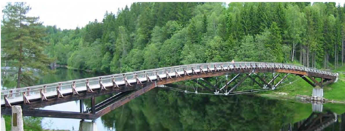
Fig. 15.3 Footbridge at Lardal, Norway (photo: A. Rönquist)
