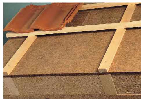
Utilisation of fibreboard in a roof construction
