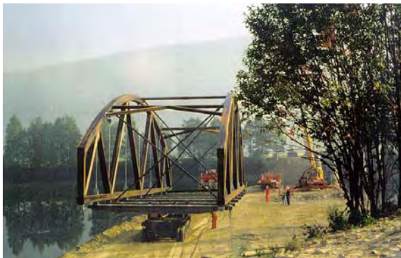
Fig. 15.18 Erection of Evenstad bridge in 1996 (photo: Moelven Limtre AS)
