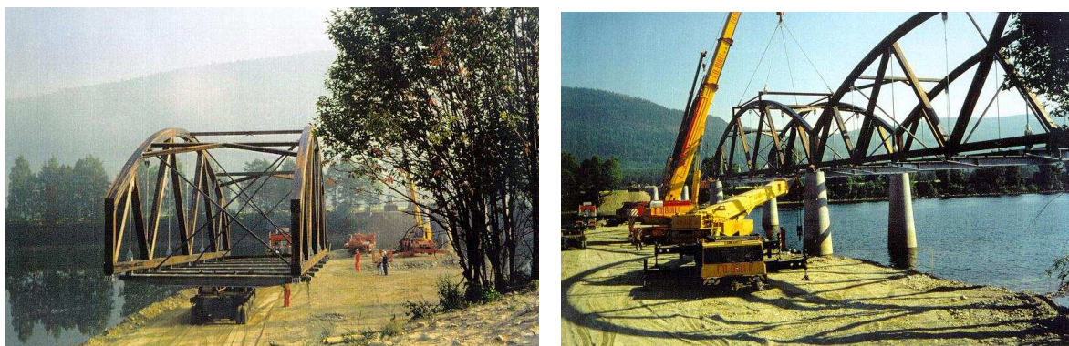
Fig. 17 Erection of Evenstad bridge in 1996 (photo: Moelven Limtre AS)
