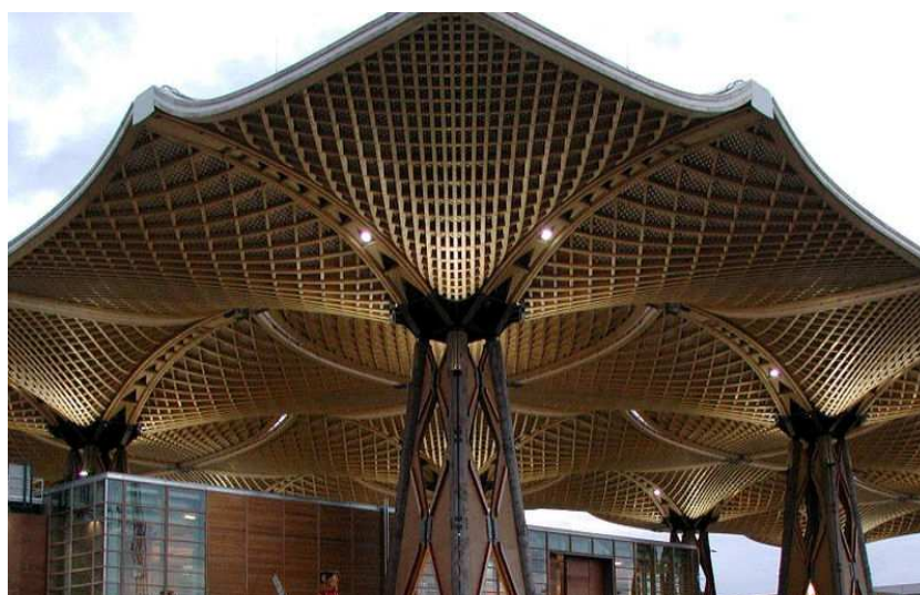
Fig. 7 Pavilion covering - EXPO 2000 in Hannover (z: internet)
