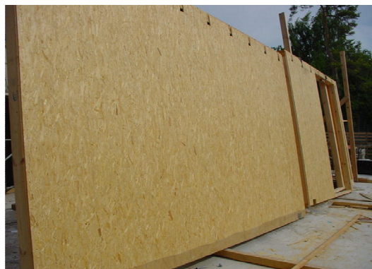
Fig. 3 OSB and its utilisation as load-carrying sheathing material in a shear -wall
