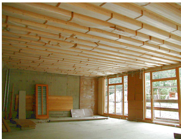
Fig. 34 Ribbed plate and boxed cross-sections built-up with CLT-elements
