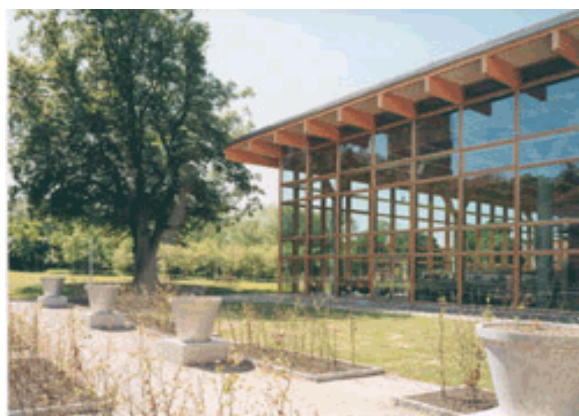
Fig. 8 Glulam beams in a library in Sweden (Reproduced by permission of Svenskt Limträ AB)
