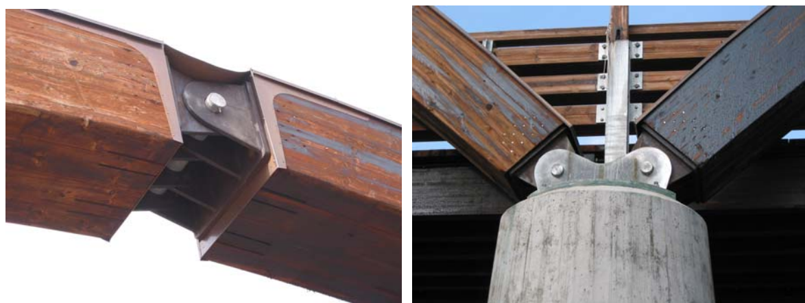
Obr. 14 – Detaily mosta Tynset (Foto: K. Bell)
