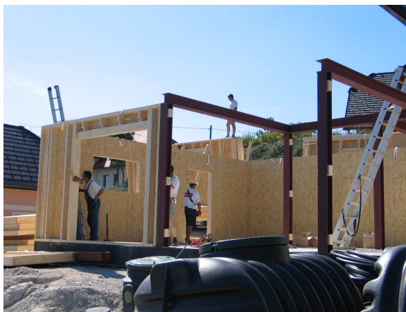
Fig. 12. Reinforcement of the timber structure with the steel frames.
