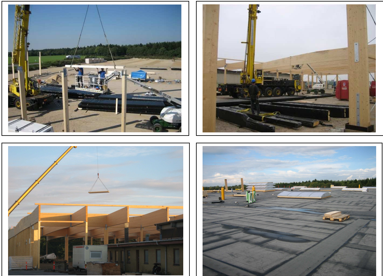
Fig. 4 Erection of the building
