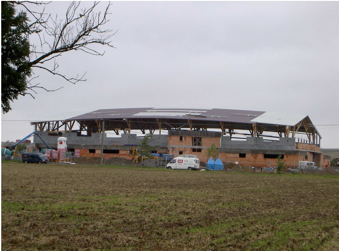
Fig. 8 Erection of the roof
