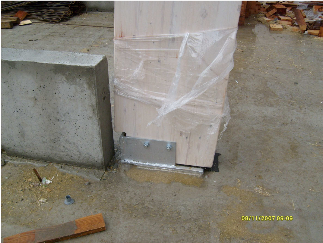
Fig. 16 Detail of timber arch anchoring
