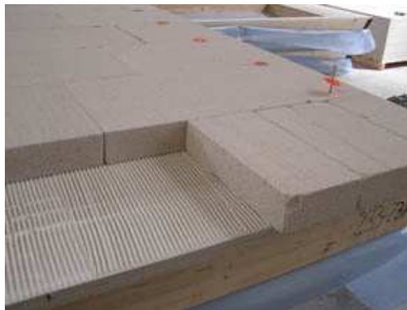
Pic. 3 Glueing of Multipor
