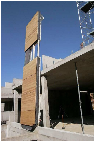
Fig. 6 First erected wall element of the office “towers”
