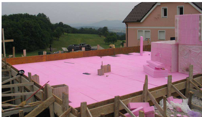
Fig. 11. 20 cm of the XPS thermal insulation in the foundation floor - plate.
