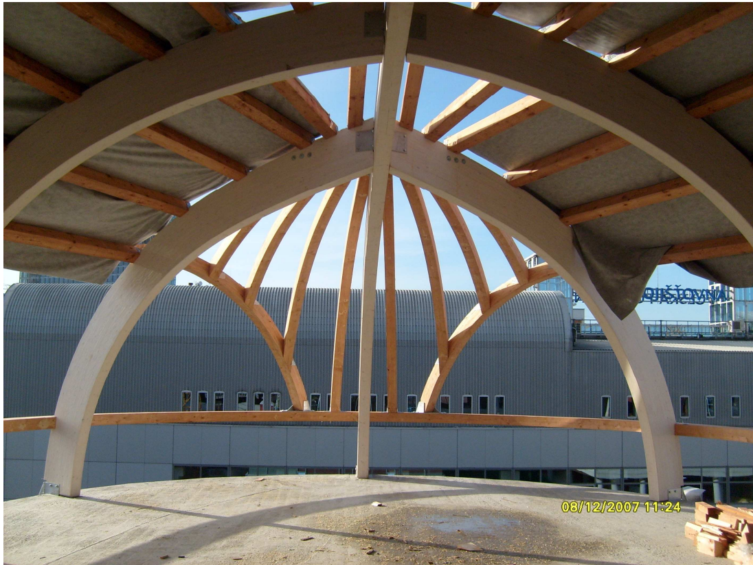
Fig. 8 Erection of the roof
