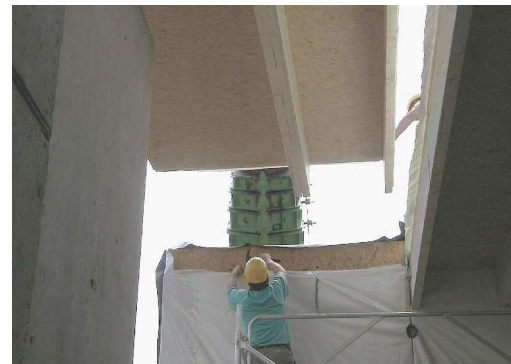
Fig. 10 Assembling of the roof elements above the office
