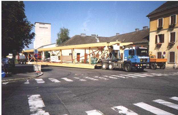
Fig. 5 Transportation of the bridge
