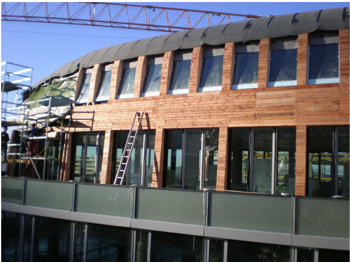
Fig. 13 Erection of the roof
