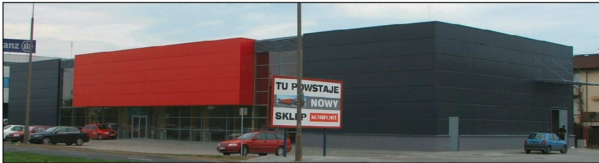
Fig. 5 The building facade
