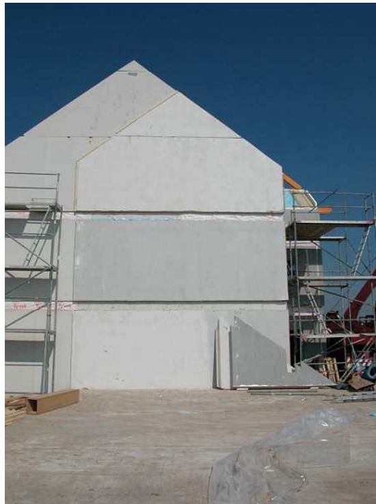
Pic. 4 Gable wall with Multipor
