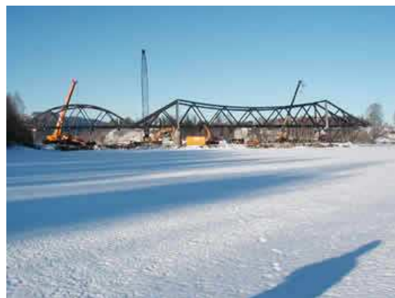
Fig. 6 Lifting of the truss
