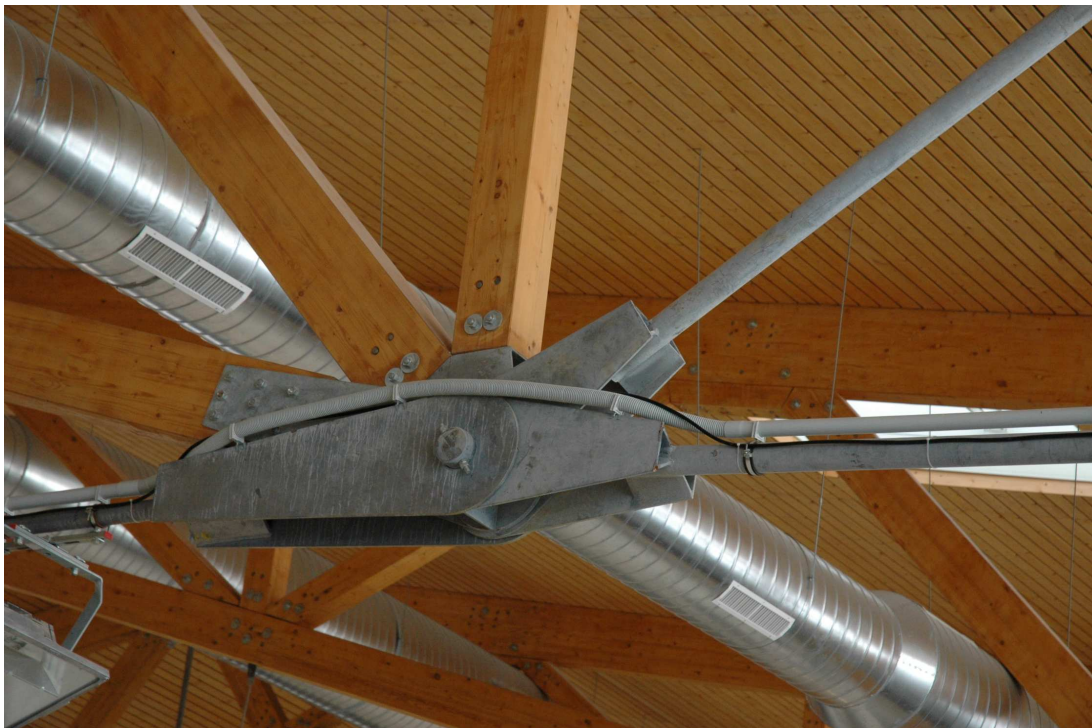
Fig. 10 Detail of timber - steel bars joint
