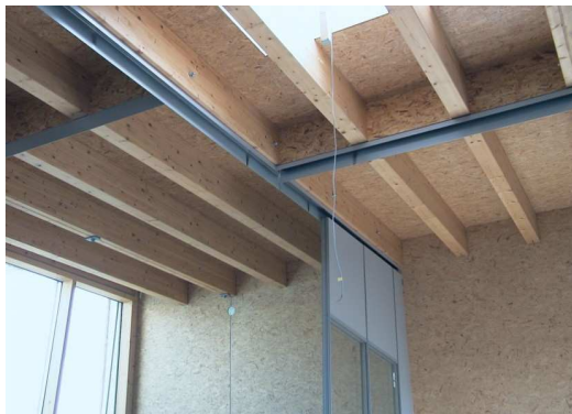
Fig. 9 Roof above the offices (with parts of the interior walls)
