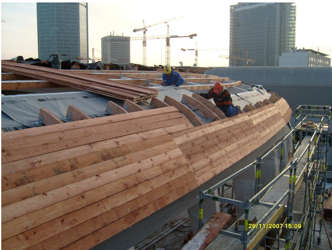
Fig. 11 Erection of the roof
