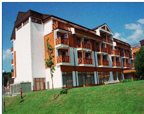
Fig. 1: Photo of the hotel from the east side.
