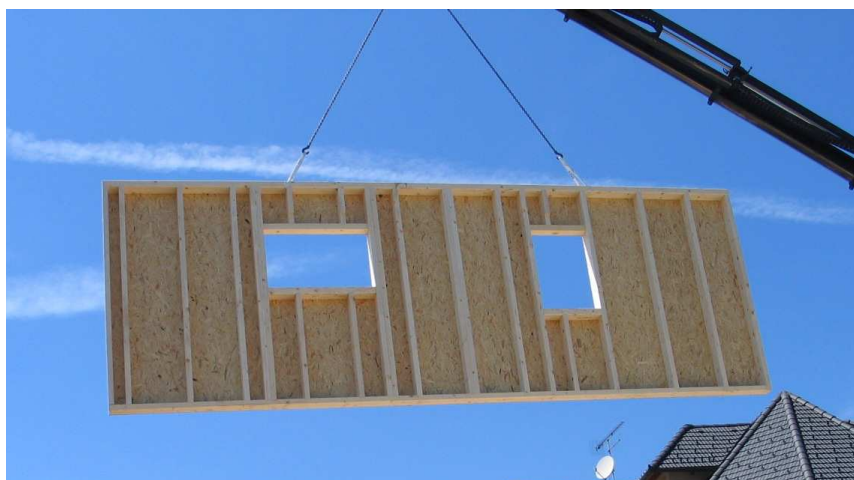
Fig. 3. Load carrying wall.
