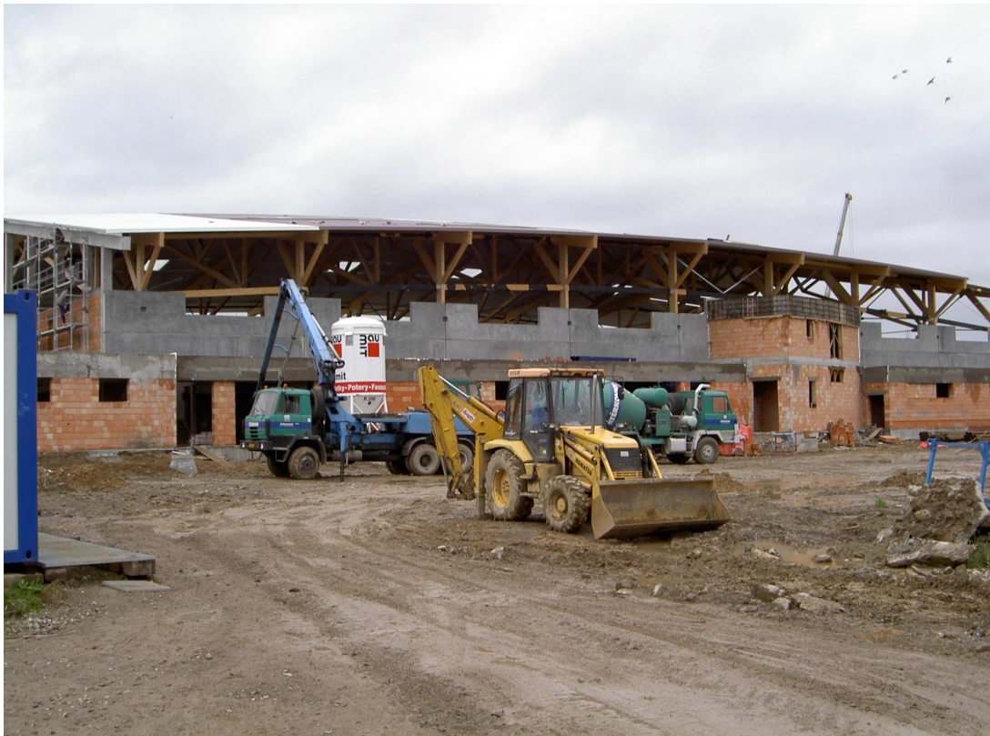
Fig. 9 Erection of the bearing system
