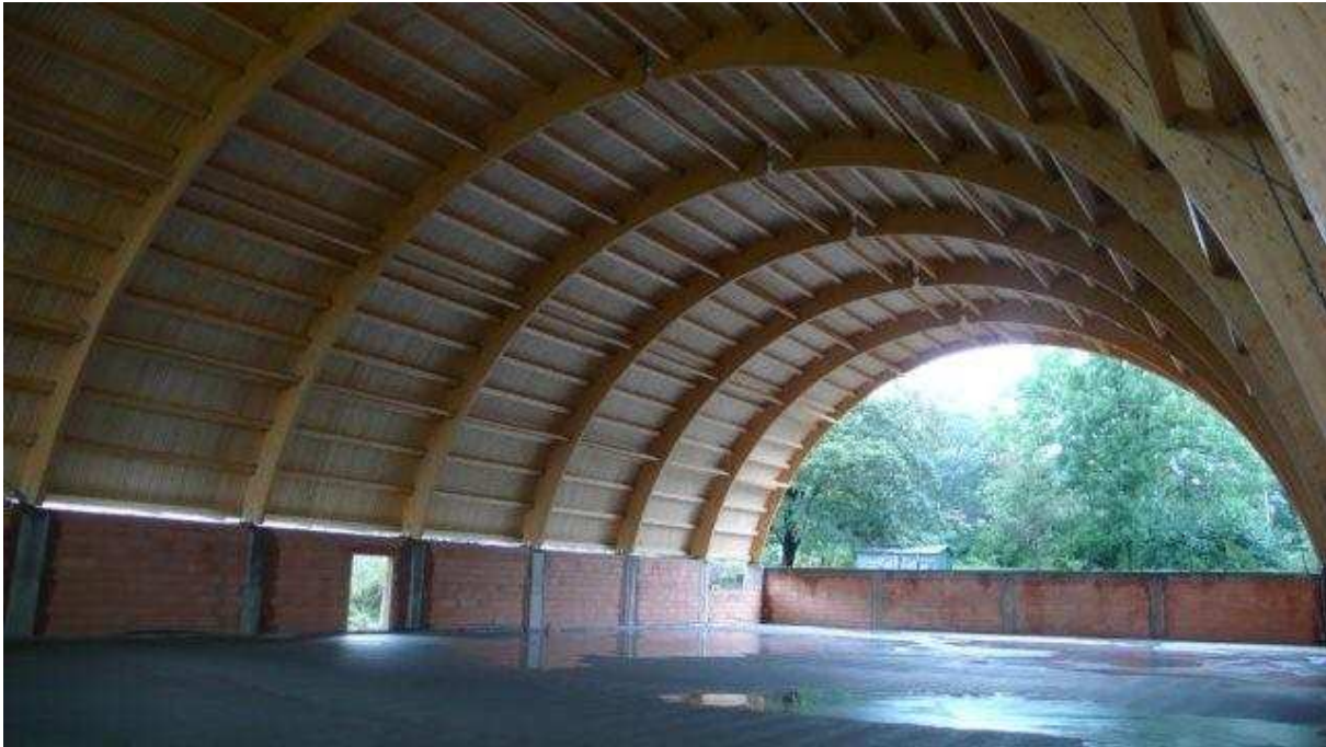
Fig. 7 Roofed sports hall with external filling masonry
