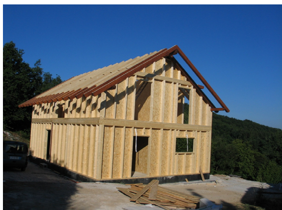
Fig. 13. Placed and fixed load carrying elements (left). Covered and closed building with the facade plates (right).
