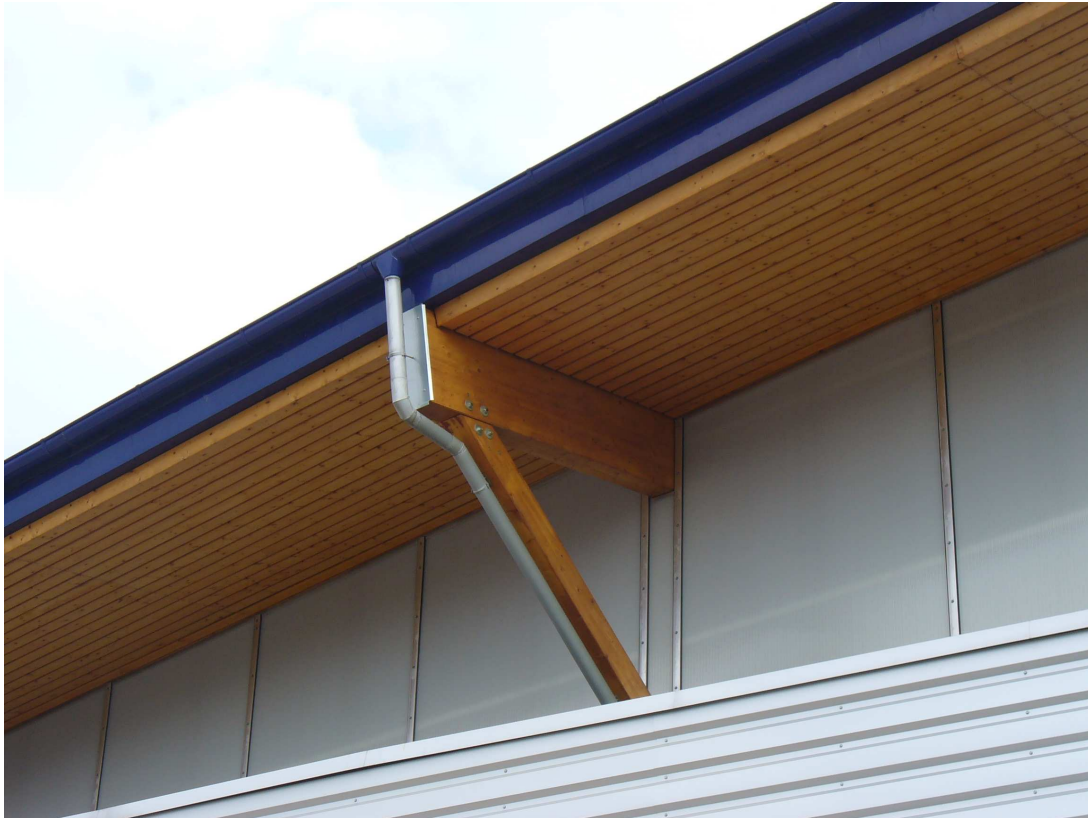
Fig. 11 Detail of protecting timber parts against weathering
