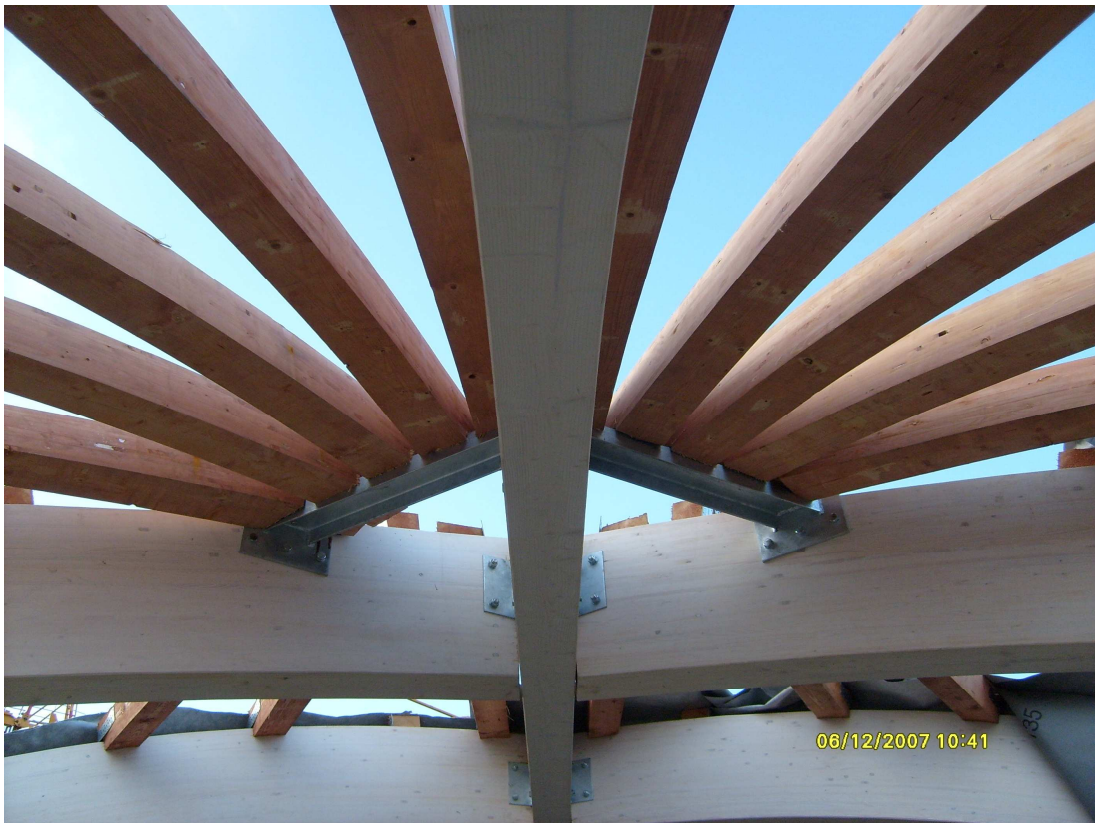
Fig. 17 Detail of timber to timber joints
