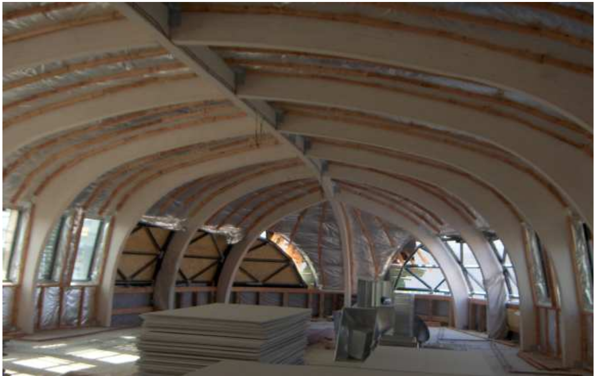
Fig. 12 Erection of the roof
