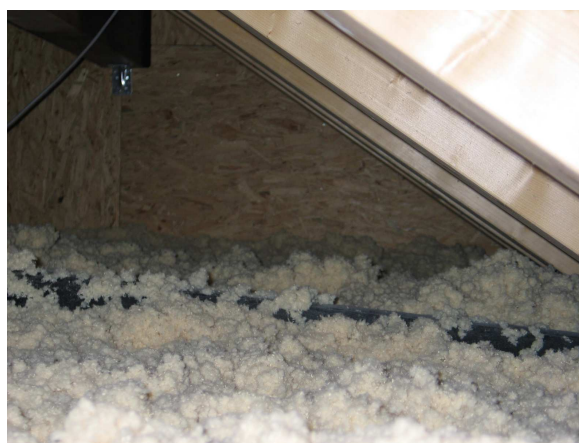
Fig. 14. Filling the blown-in wood fiber insulation.
