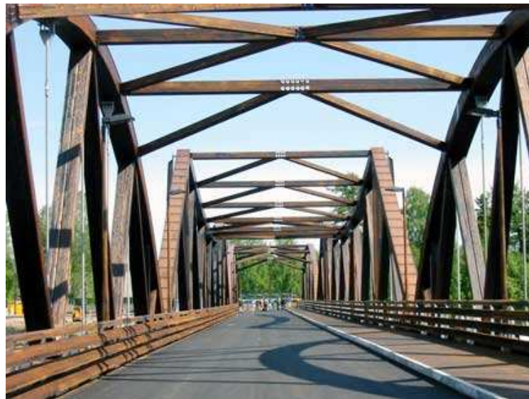
Fig. 7 View of the new Flisa bridge
