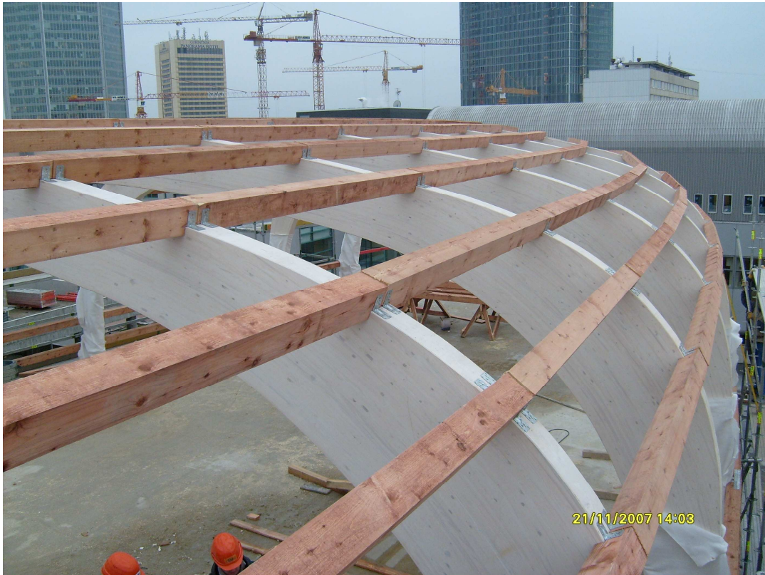
Fig. 10 Erection of the roof
