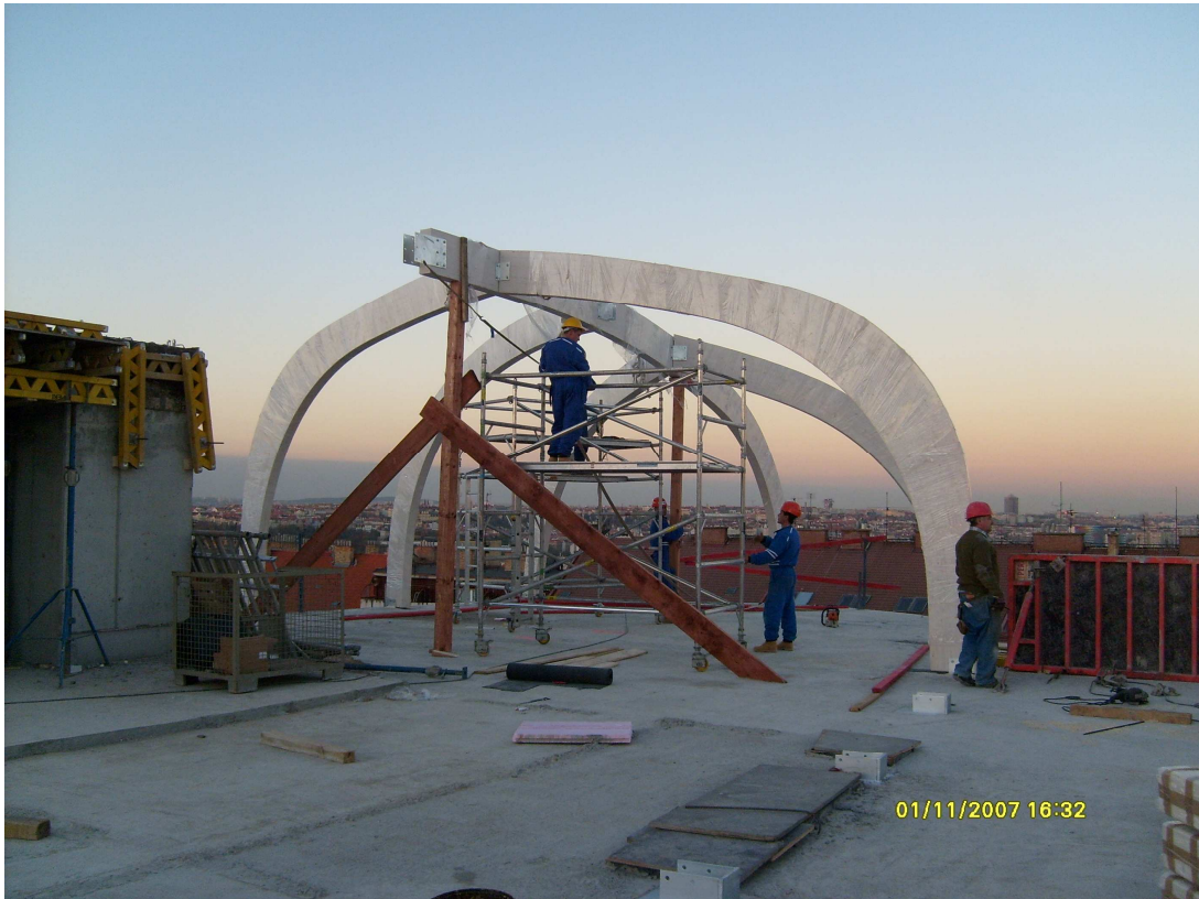
Fig. 6 Erection of the roof
