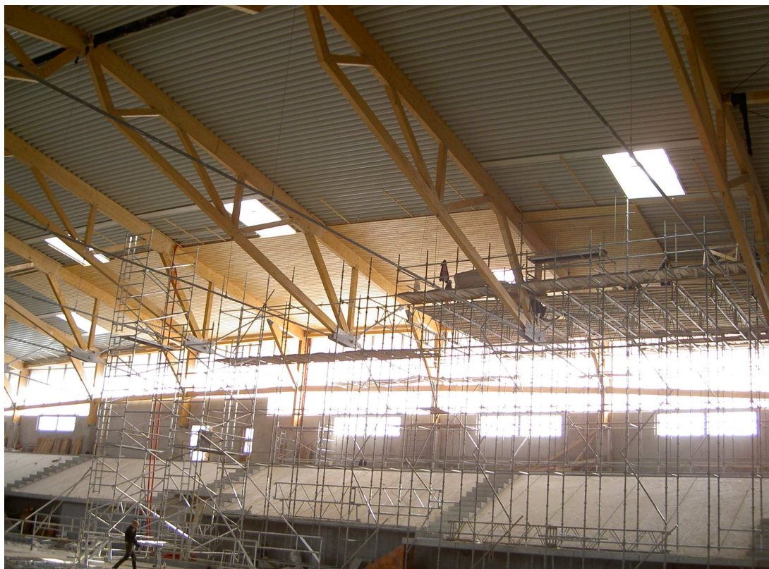
Fig. 6 Erection of the roof
