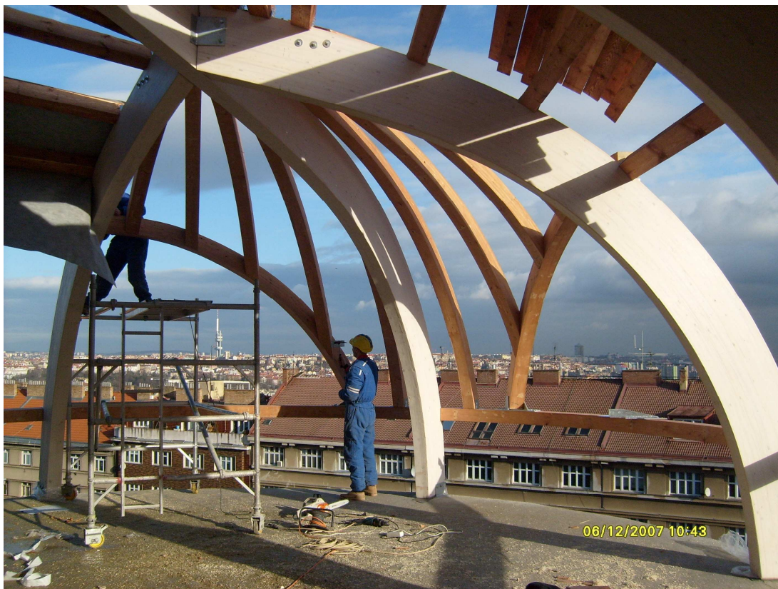
Fig. 7 Erection of the roof
