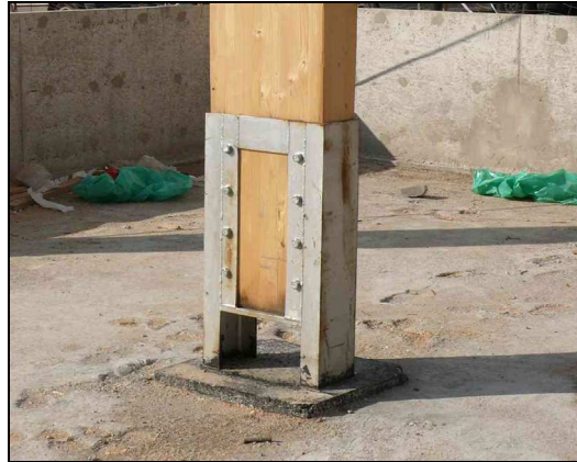
Fig. 3 Column support joint
