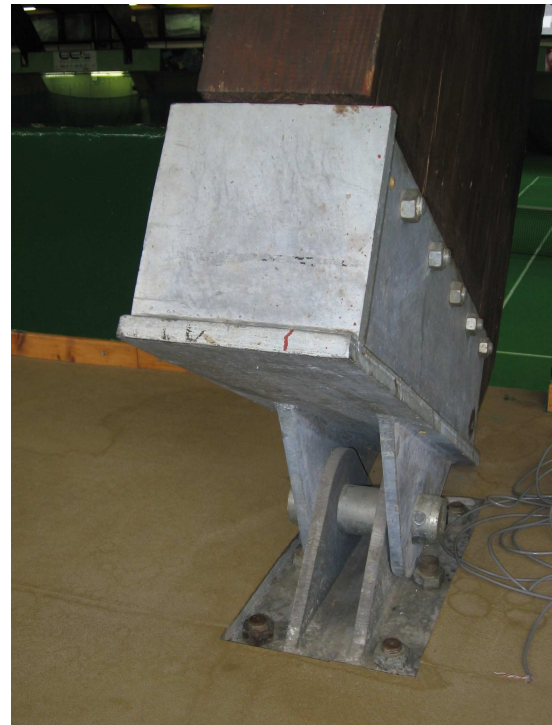
Fig. 10: Connection of the main timber element to the concrete foundation.
