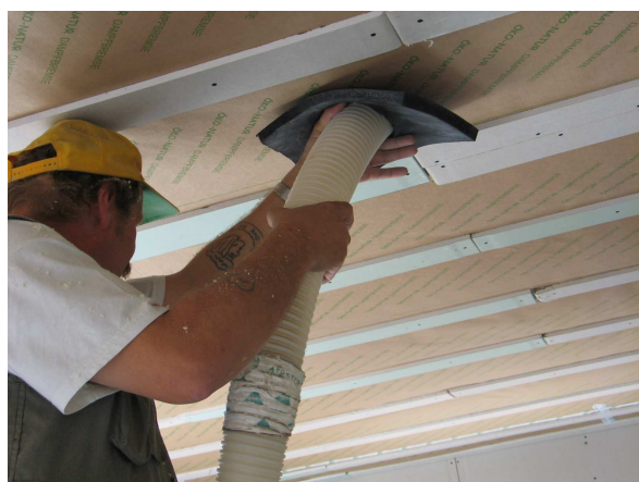
Fig. 14. Filling the blown-in wood fiber insulation.
