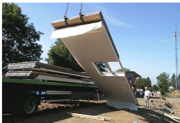
Fig. 14 Lifting of a wall element by means of a mobile-crane
