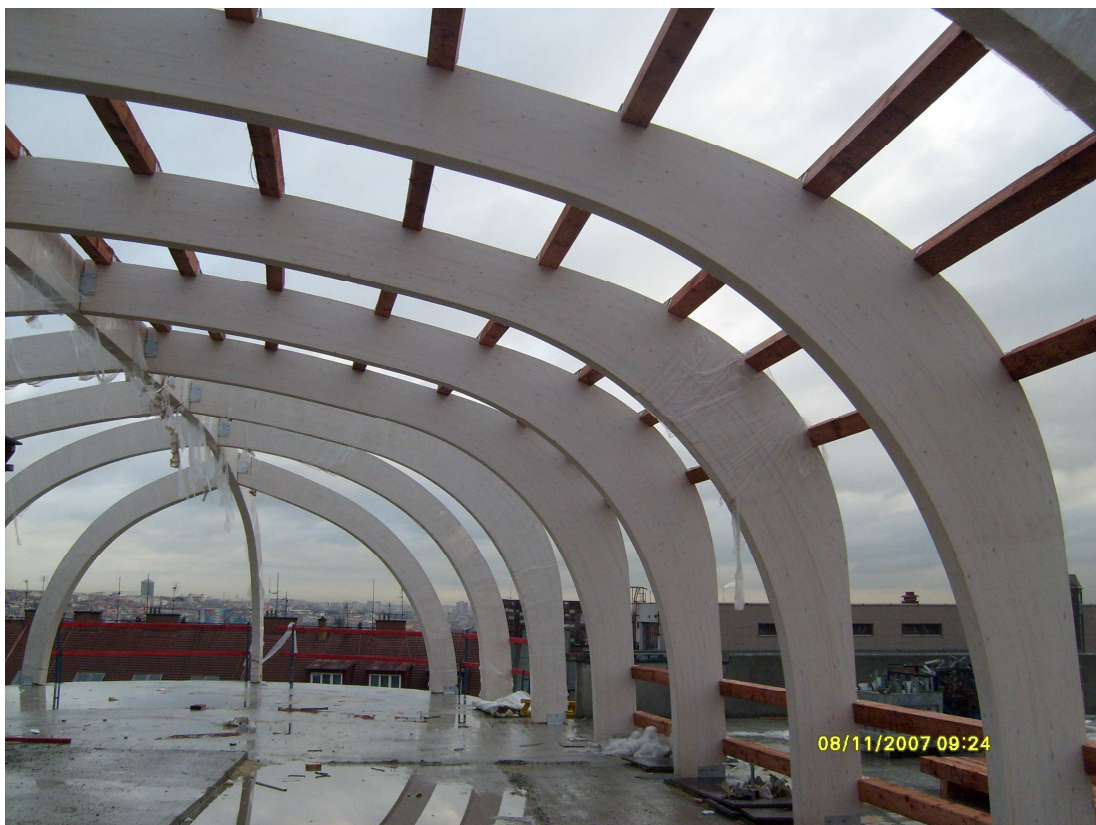
Fig. 9 Erection of the roof
