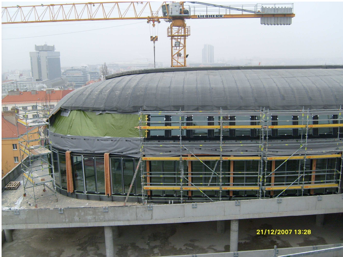
Fig. 14 Erection of the roof
