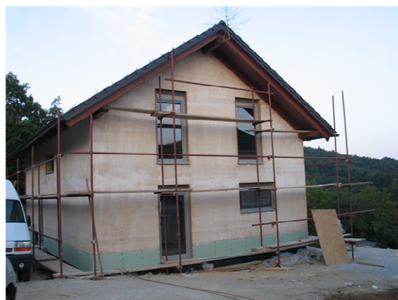
Fig. 13. Placed and fixed load carrying elements (left). Covered and closed building with the facade plates (right).
