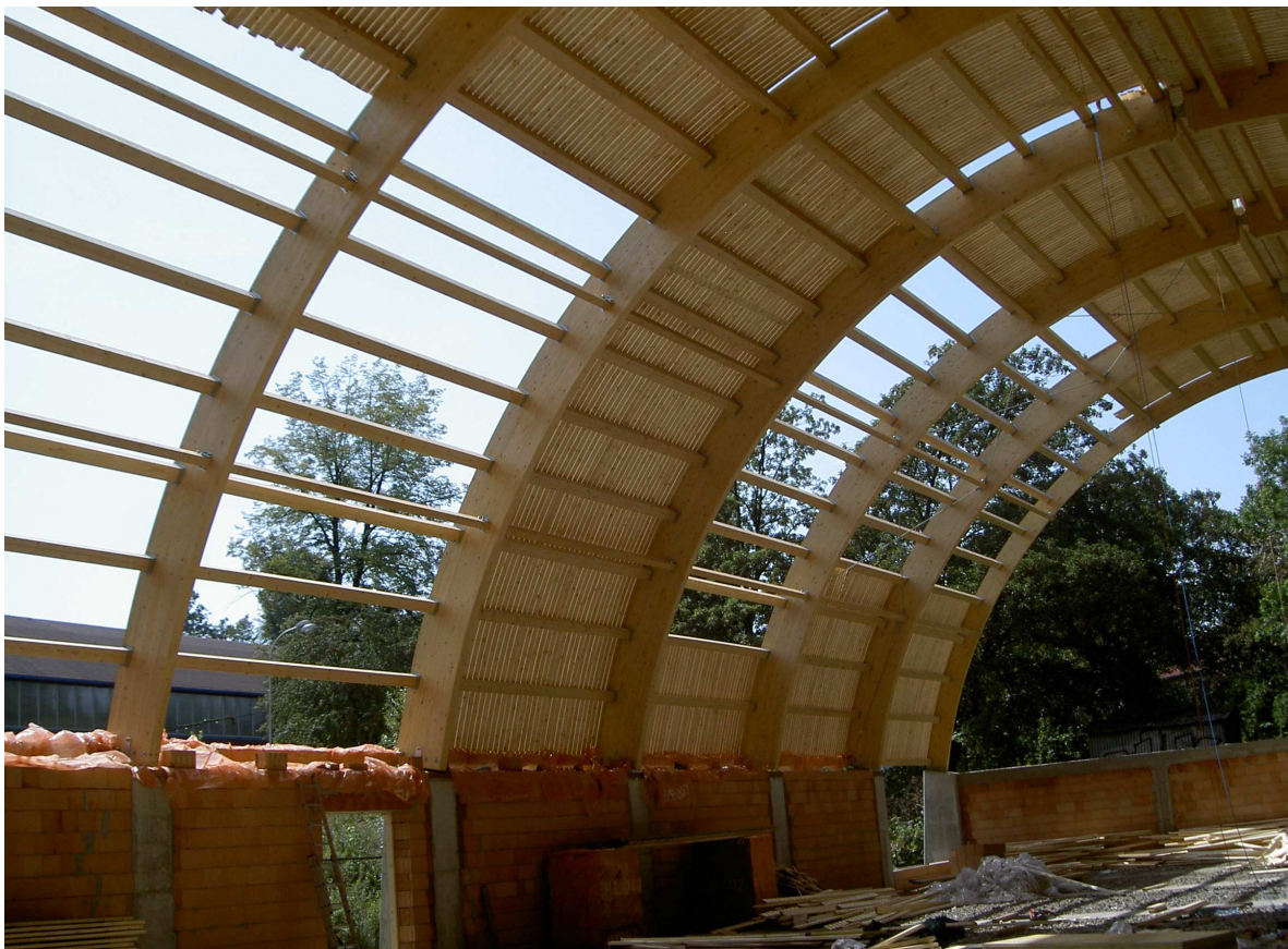
Fig. 5 Gradual roofing of the soffite
