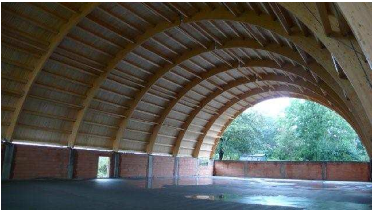
Fig. 7 Roofed sports hall with external filling masonry
