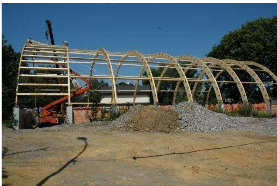
Fig. 3 Setting of the purlins into BOVA straps between glue laminated arches
