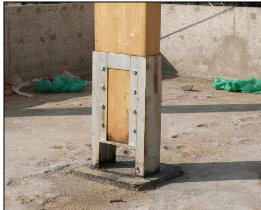
Fig. 3 Column support joint
