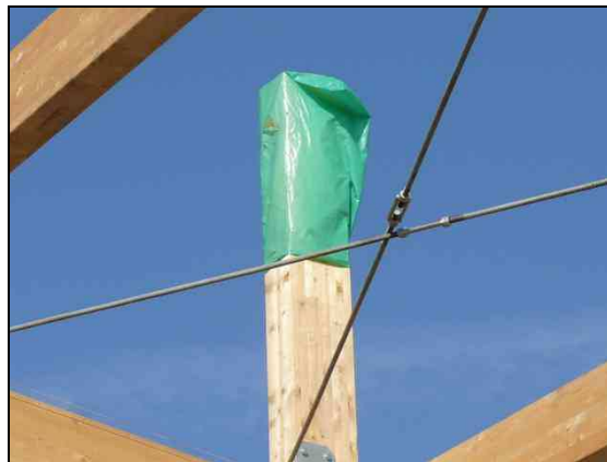
Fig. 11 Weather dumping protection of a column element
