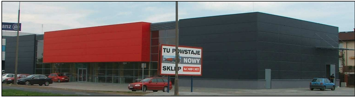
Fig. 5 The building facade
