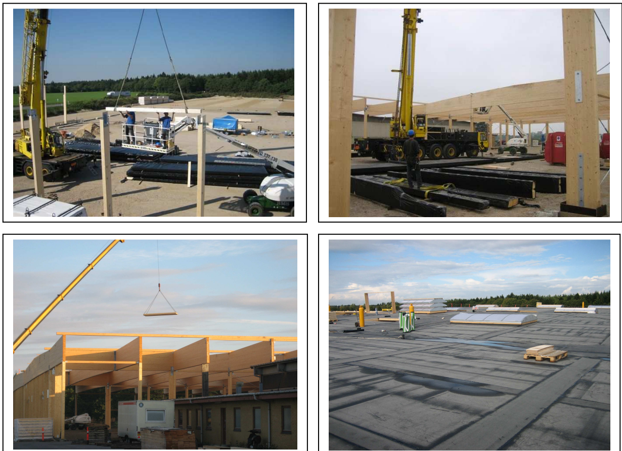
Fig. 4 Erection of the building
