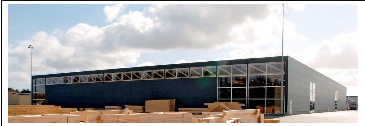
Fig. 1 The building seen from the north
