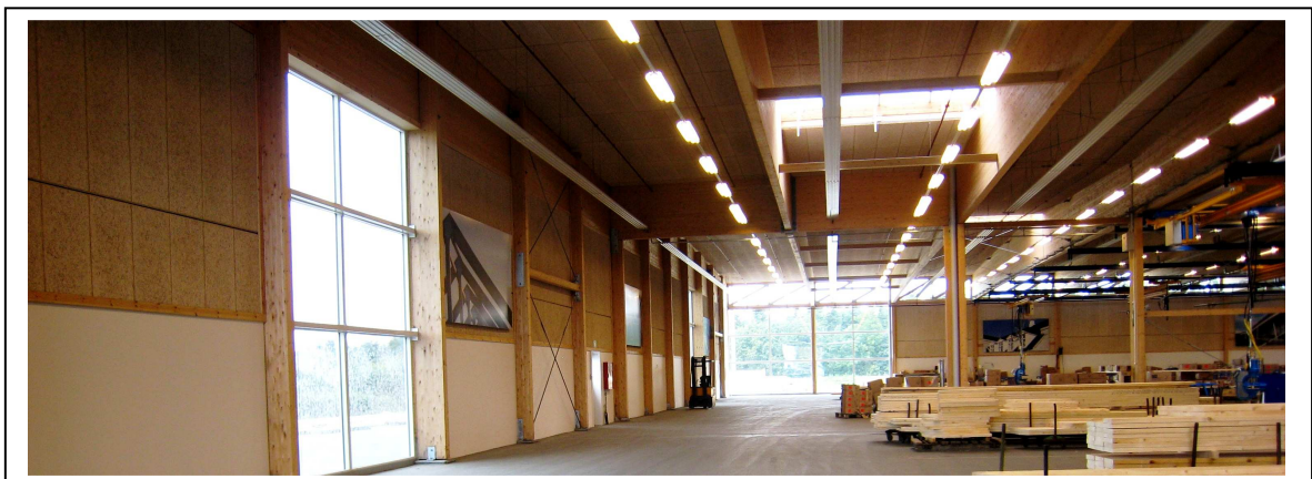
Fig. 2 The building seen from the inside
