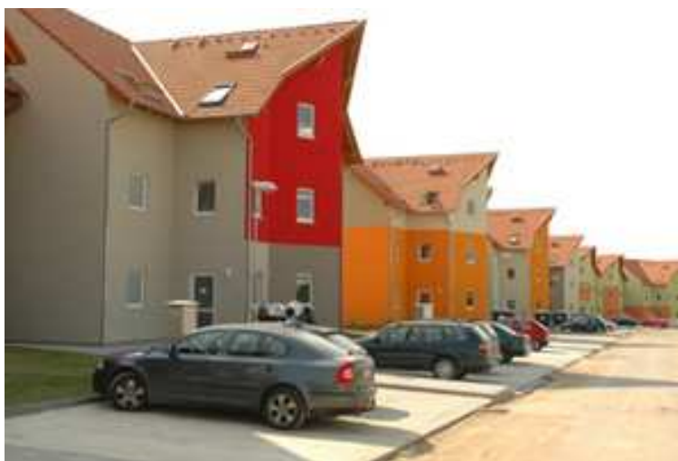
Pic. 1 Apartment houses in Chýně
