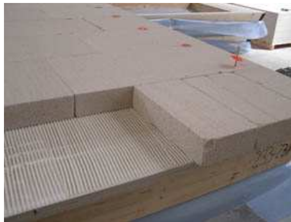
Pic. 3 Glueing of Multipor
