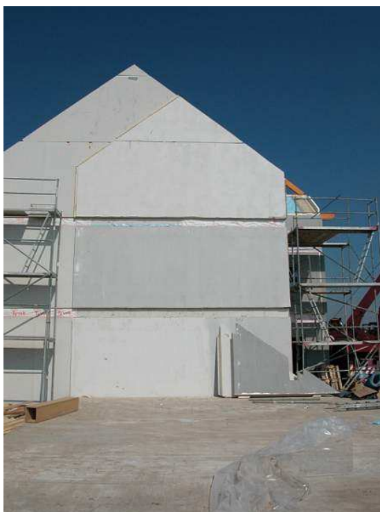
Pic. 4 Gable wall with Multipor
