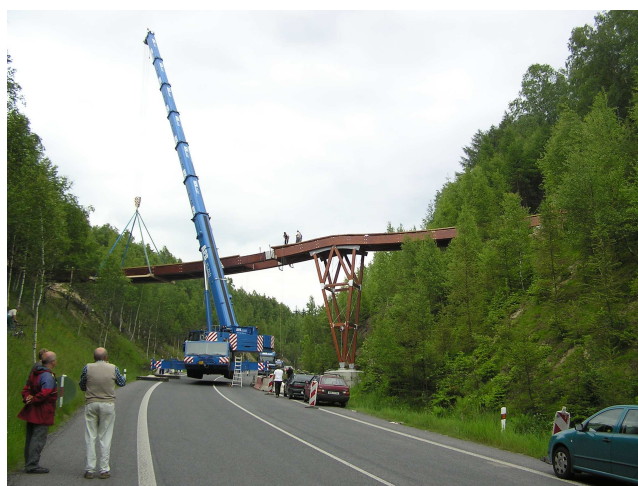
Fig. 5 Bridge erection sequence
