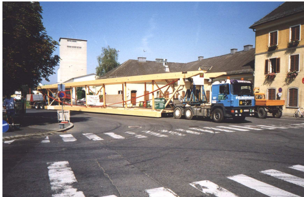
Fig. 5 Transportation of the bridge
