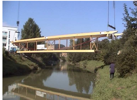
Fig. 6 Assembly of the bridge
