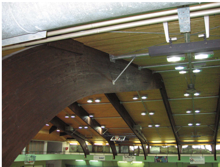
Fig. 11: A steel bracing system in the upper horizontal beam plane.
