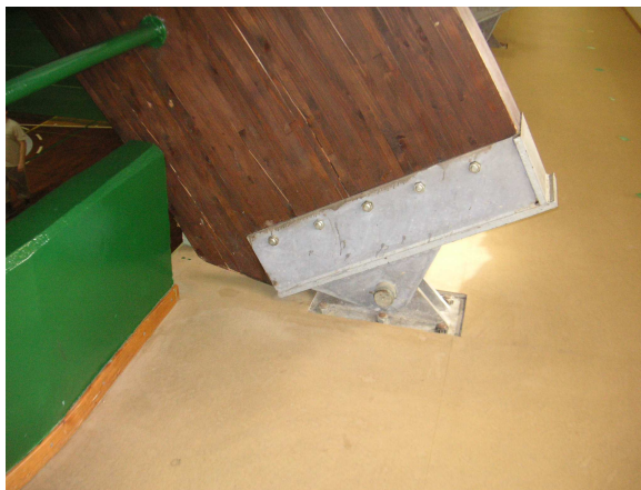
Fig. 13: Cracks by the connection to the base (a) and in the middle hinge (b).
