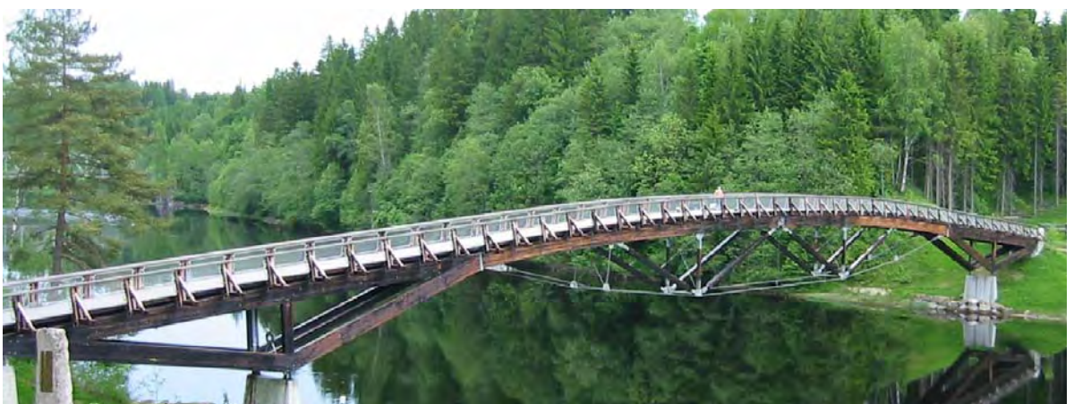
Fig. 3 Footbridge at Lardal, Norway (photo: A. Rönquist)
