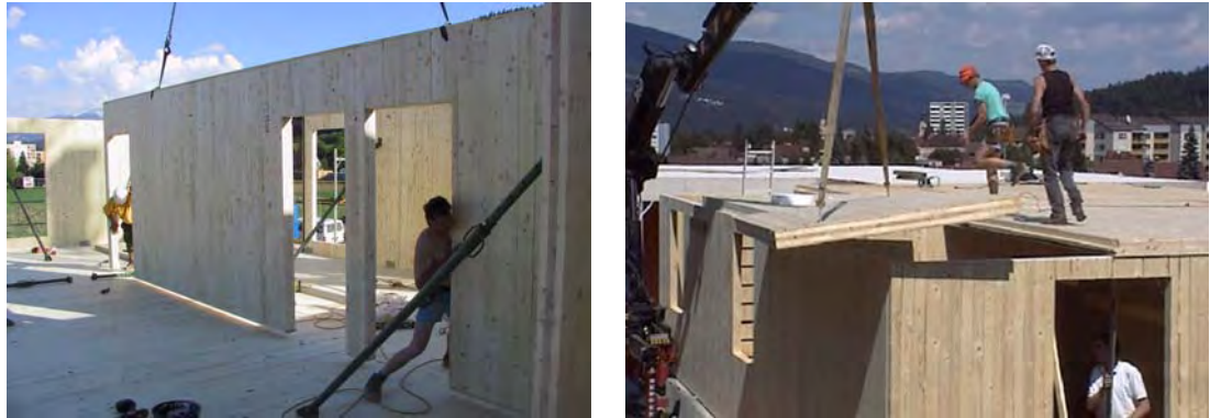
Fig. 30 Unfinished building: Erection of walls, lifting of floors
