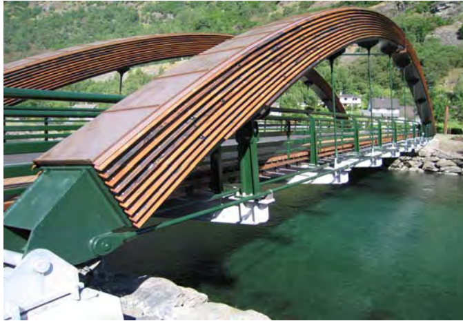
Fig. 17 Fretheim bridge at Flåm in western Norway (photo: R. Abrahamsen, SWECO Grøner AS)
