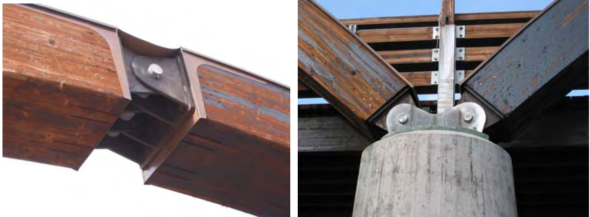
Fig. 14 Details of the Tynset bridge (photo: K. Bell)
