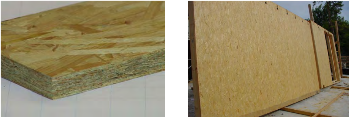
Fig. 3 OSB and its utilisation as load-carrying sheathing material in a shear -wall
