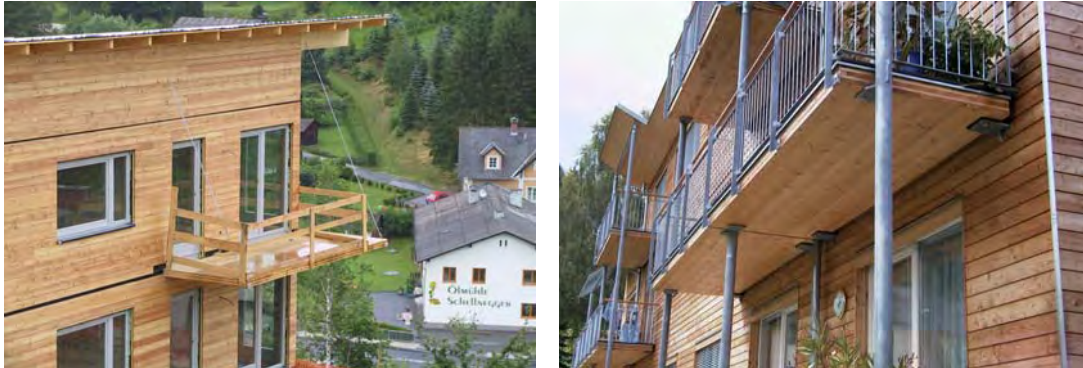
Fig. 34 Cantilever and point-bearing balcony plates
