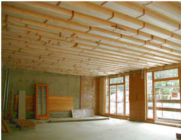
Fig. 35 Ribbed plate and boxed cross-sections built-up with CLT-elements
