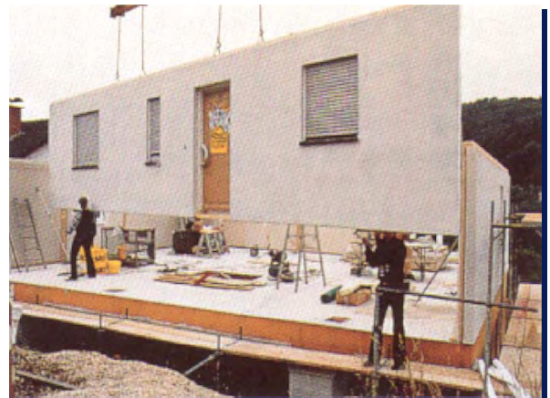
b. Mounting of walls on the building-site
