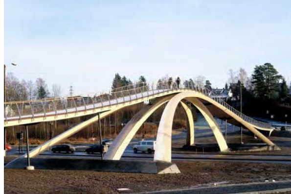
Fig. 5 Leonardo da Vinci Bridge in Ås, Norway (Reproduced by permission of the Norwegian Public Roads Administration)
