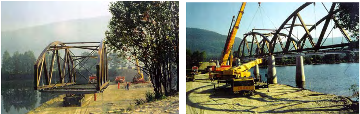
Fig. 18 Erection of Evenstad bridge in 1996 (photo: Moelven Limtre AS)
