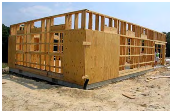
Fig. 6 9-layered plywood (robinia) and the use of plywood as stiffening elements in a shear-wall
