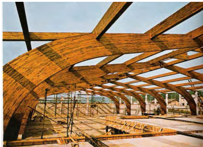
Fig. 3 Example of a glulam arch
