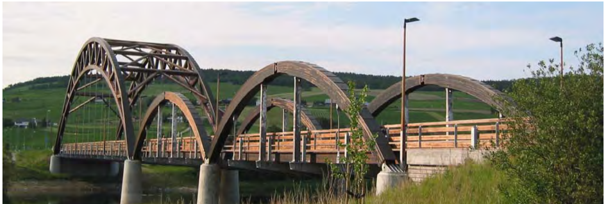
Fig. 6 Tynset bridge, Norway (photo: K.Bell)
