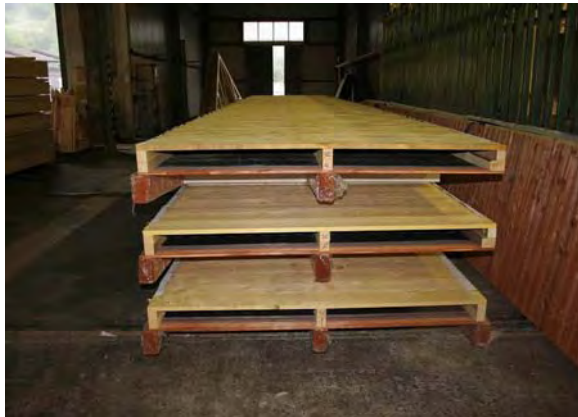
a. Prefabricated roof beams with boards
