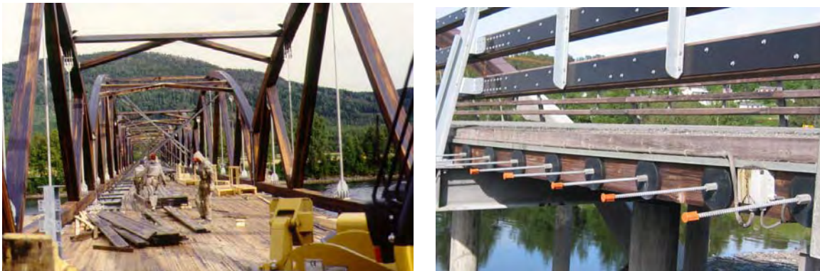
Fig. 12 Laying the deck of Evenstad bridge (photo: Moelven Limtre) and detail of Måsør bridge (photo: K. Bell)
