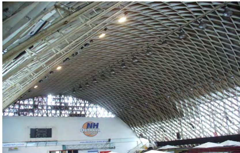
Fig. 1 Lamellar vault of the sports hall roof
