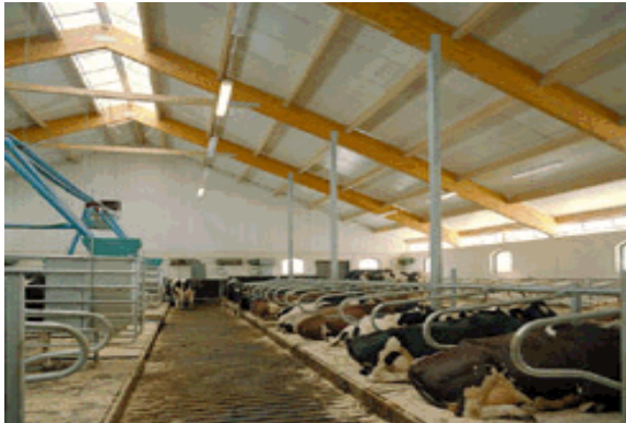
Fig. 10 Three-pin frame in a barn in Sweden (Reproduced by permission of Svenskt Limträ AB)
