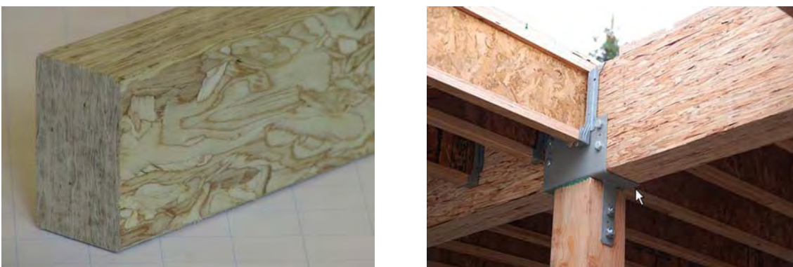
Fig. 4 LSL and their use as beams
