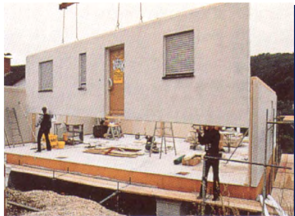
b. Mounting of walls on the building-site
