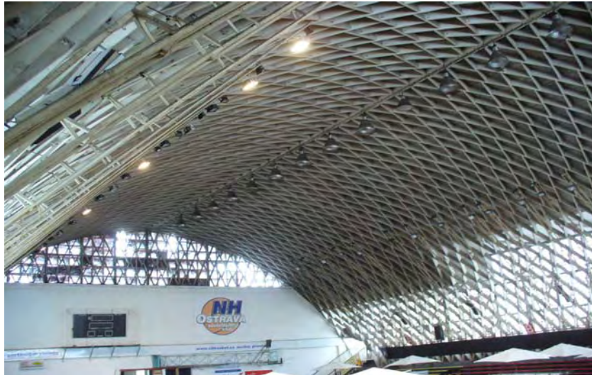
Fig. 1 Lamellar vault of the sports hall roof
