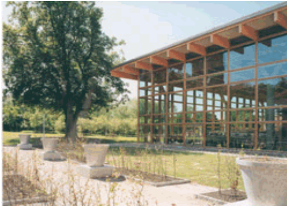
Fig. 8 Glulam beams in a library in Sweden (Reproduced by permission of Svenskt Limträ AB)
