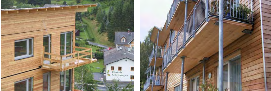
Fig. 33 Cantilever and point-bearing balcony plates
