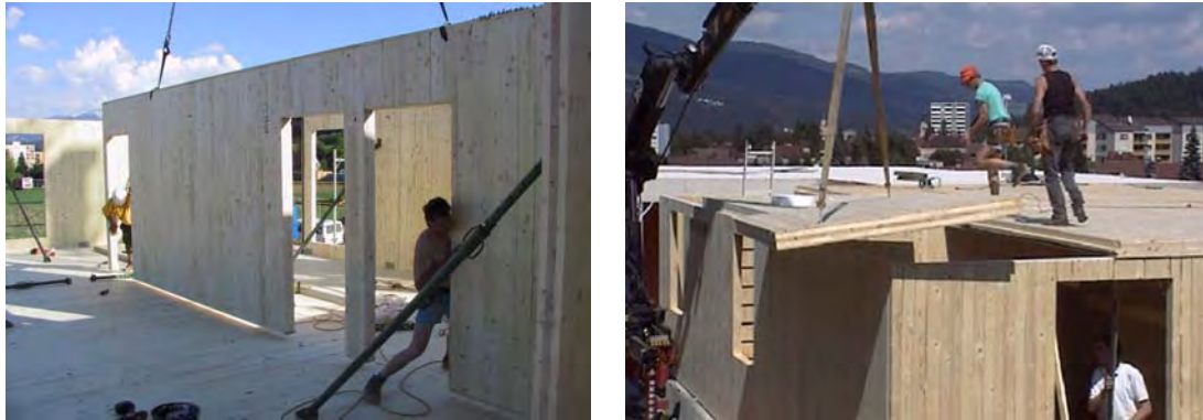
Fig. 29 Unfinished building: Erection of walls, lifting of floors
