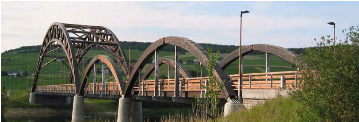
Fig. 6 Tynset bridge, Norway (photo: K.Bell)
