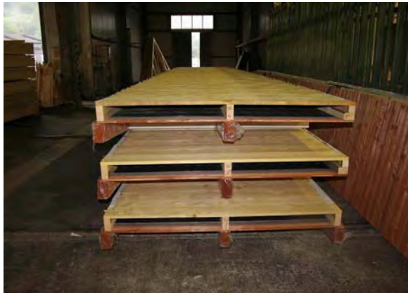
a. Prefabricated roof beams with boards
