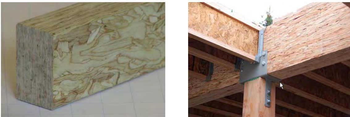
Fig. 4 LSL and their use as beams
