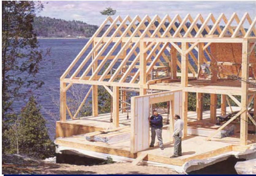
Fig. 1 Post and beam building system
