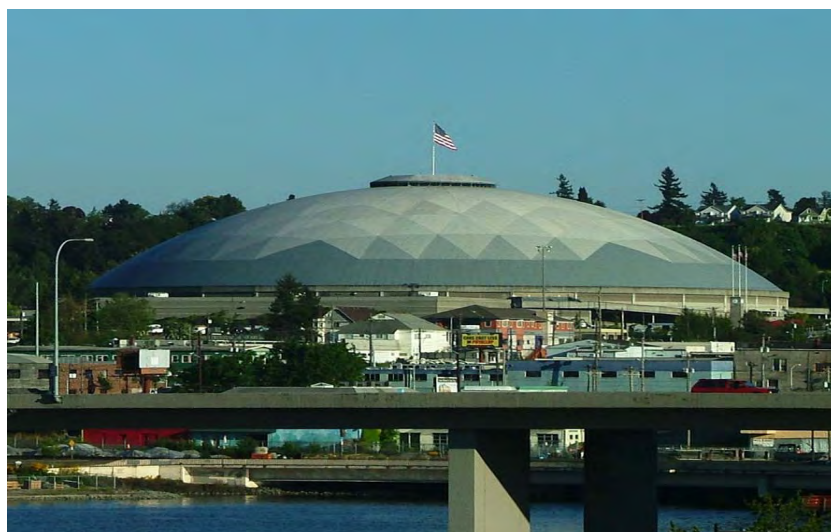
Fig. 5 Tacoma Dome in USA (source: Internet)
