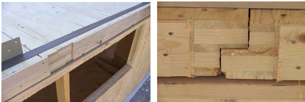
Fig. 38 Floor-floor-joint
