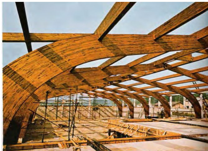
Fig. 3 Example of a glulam arch
