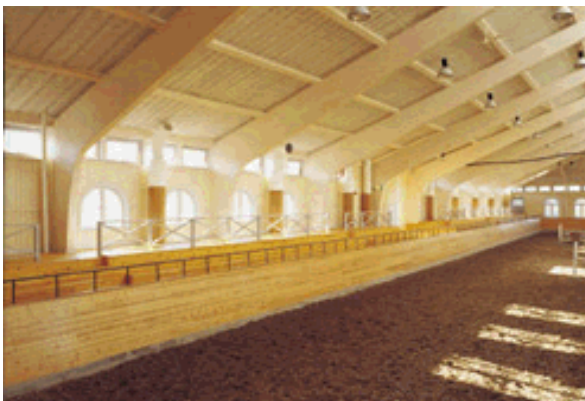
Fig. 12 Portal frame in a riding school in Sweden (Reproduced by permission of Svenskt Limträ AB)
