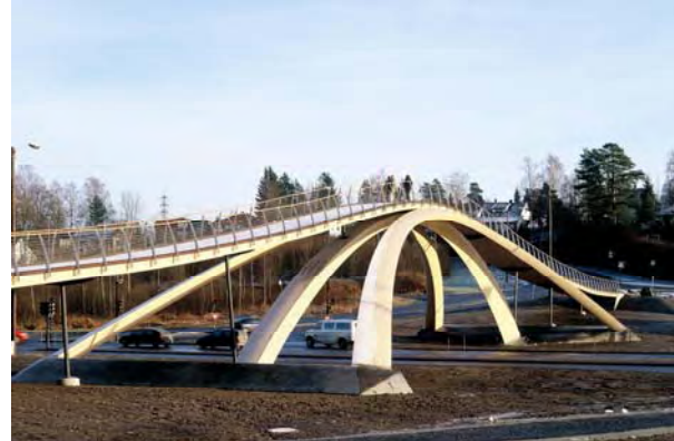
Fig. 5 Leonardo da Vinci Bridge in Ås, Norway (Reproduced by permission of the Norwegian Public Roads Administration)
