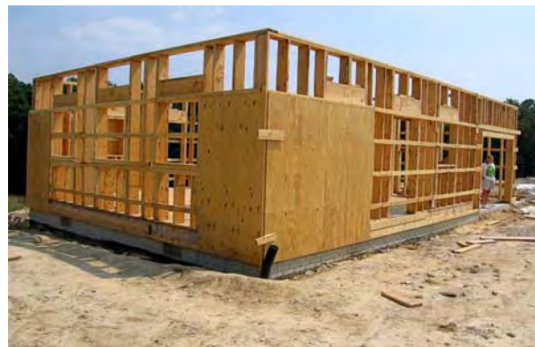
Fig. 6 9-layered plywood (robinia) and the use of plywood as stiffening elements in a shear-wall
