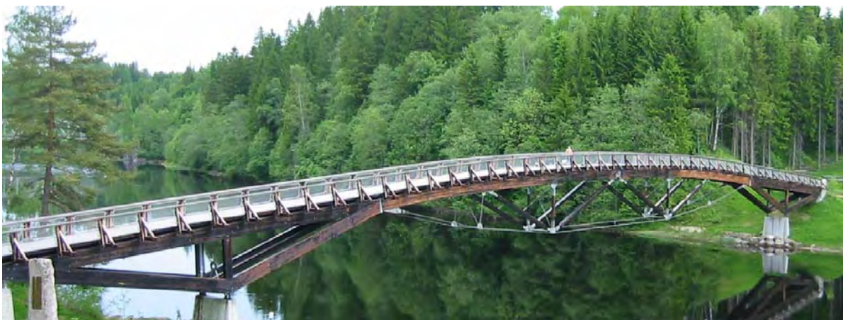
Fig. 3 Footbridge at Lardal, Norway (photo: A. Rönquist)
