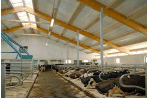
Fig. 10 Three-pin frame in a barn in Sweden (Reproduced by permission of Svenskt Limträ AB)
