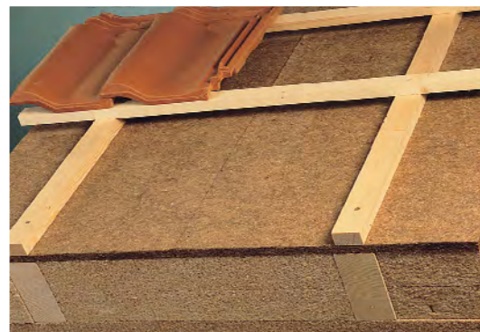
Utilisation of fibreboard in a roof construction
