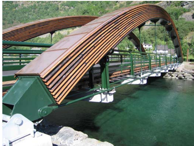
Fig. 17 Fretheim bridge at Flåm in western Norway (photo: R. Abrahamsen, SWECO Grøner AS)
