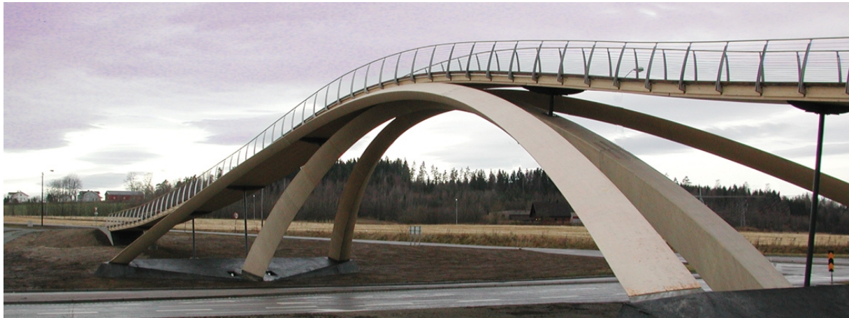
Fig. 2 The Leonardo footbridge at Ås, south of Oslo, Norway (photo: Moelven Limtre AS)
