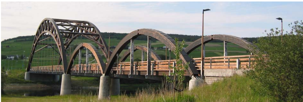
Fig. 6 Tynset bridge, Norway (photo: K.Bell)
